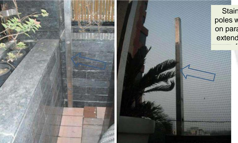
Stainless steel poles were erected on parapet walls to extend foundation
