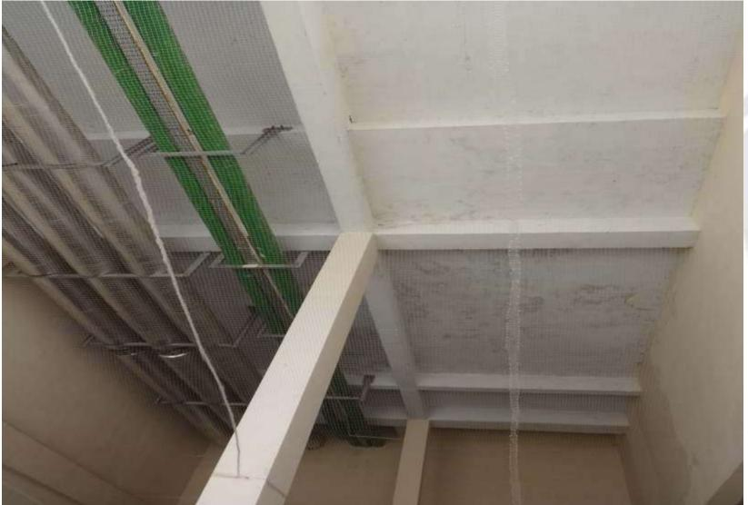
Barricading Pigeon Entry in Shaft and Duct areas
