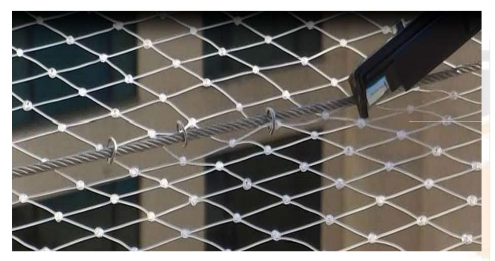
Imported Stainless Steel Rings are used to staple net with SS Rope
